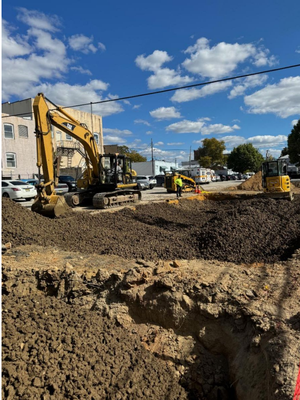
Vineland stormwater tree pit construction, October 2024 [Photo credit: Roy Messaros]
